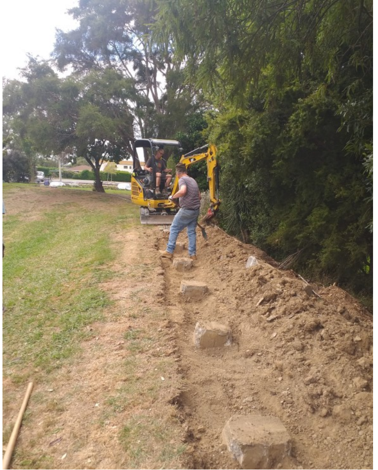
Owen Mudgway and Lawrence Brooshooft excavating the cut. Photo Jon Mason
