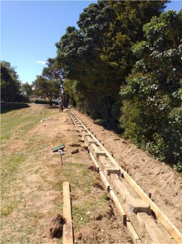
Formwork positioned for new vertical alignment Photo Jon Mason
