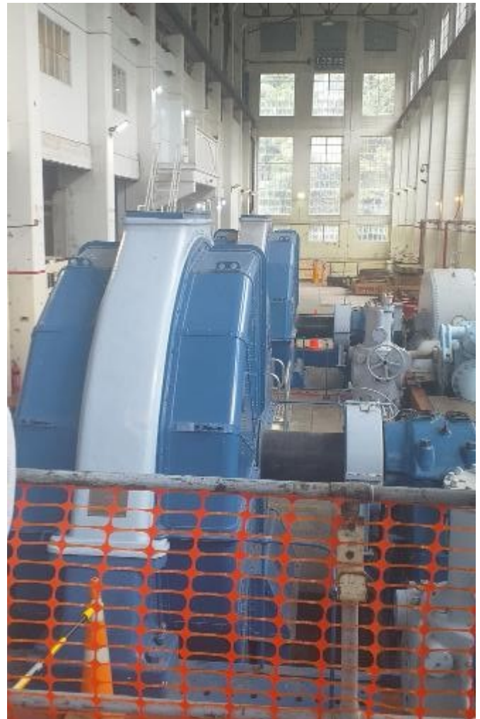
The 2 remaining 1924 Pelton Wheel Generators
