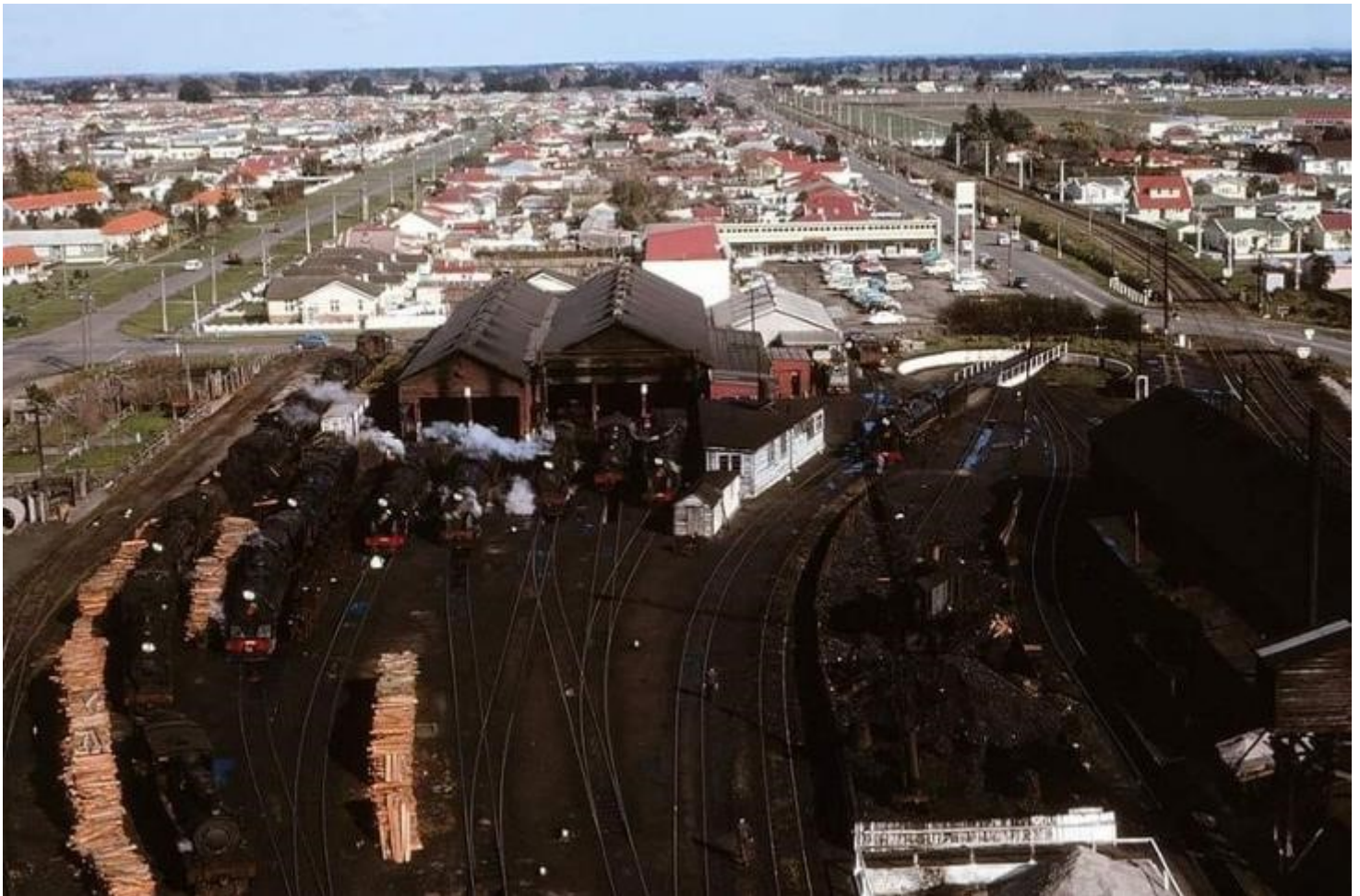
A view looking west showing Roly's work place in 1963 the present site of the Warehouse showing the loco shed's, turntable and the coal grabber. Of note in the foreground top right the large green field open space, present site of Monrad Intermediate School, Monrad Park and the Marriner Reserve Railway. Roly must have climbed a lighting tower to gain this photo, possibly to change a bulb! Photo Roland Penhall
