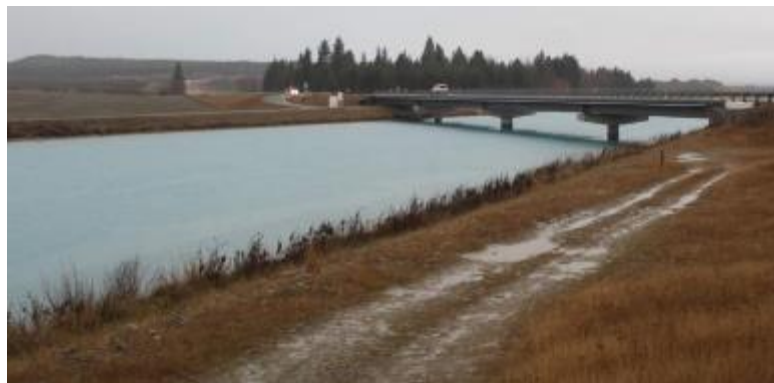
Dug in section of canal at state highway 8 crossing.
