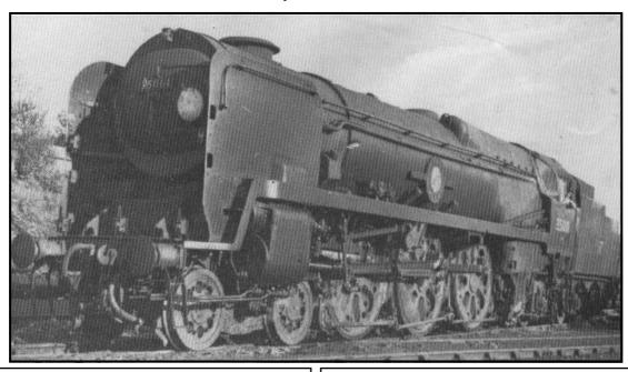
their axle loading. The large cast stretchers were gradually replaced with fabricated steel units. Further problems arose with oil leakage from the valve casing and the casing surrounding the inside connecting rod and crank. The chains driving the valve gear were found to be prone to stretching and this caused the valve timing to alter from the correct setting. Oil leaking from the enclosed cases occasionally saw a large fire burning outside the firebox.
