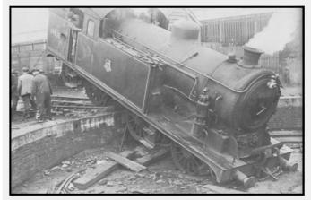
required for the tank engines operating there. However this incident took place before the pit was filled in. The driver was moving the locomotive to the nearby ash pit and failed to stop in time.
