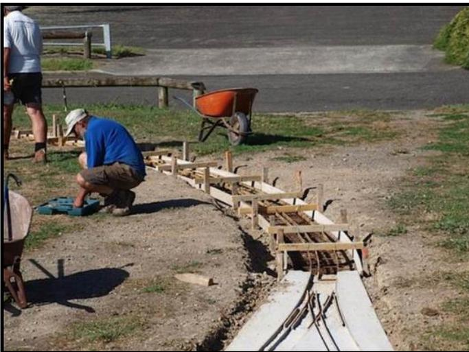
The curved track section was next boxed up and the track fabricated and welded up insitu suspended on the formwork, concrete again poured the next day.
