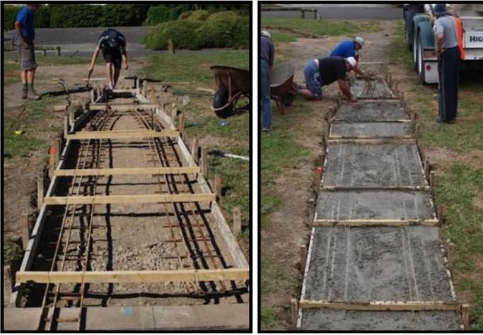
The section incorporating the Y turnout and two parallel roads was then boxed up and the prefabricated tracks and turnout were suspended and positioned on the formwork with concrete poured the next day.
