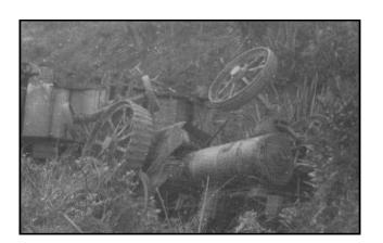
engine 'ran away' on a downhill grade. From the shape of the cylinder block I believe that the engine is a single cylinder Burrell. I don't know how the driver and steersman fared.
