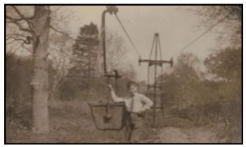
The cableway evidently brought clay from another pit to the railway where it was loaded onto the narrow gauge wagons and transported by rail to the
